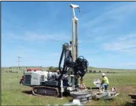
Sonic drilling rig
